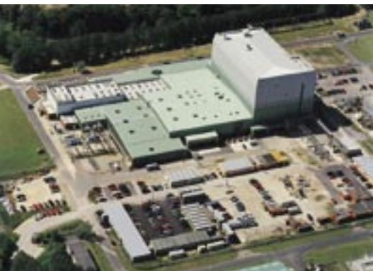
OFC one of the most advanced nuclear manufacturing plants in the world.
